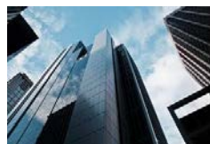
Large Commercial Office Bldg.
