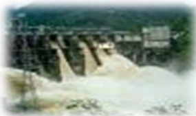
Hydro Power Plant
