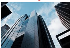
Large Commercial Office Bldg.
