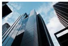
Large Commercial Office Bldg.
